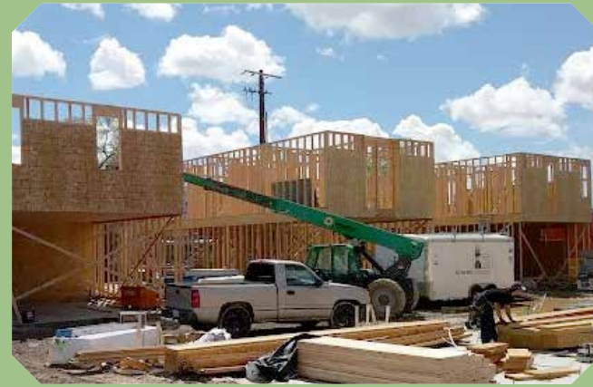
Framing goes up at the Marmalade project
